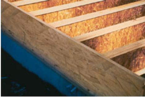
Rim boards provide basic closure and critical structural load transfer in a structure. The transfer of vertical loads includes the weight of the structure above the rim board as well as design and construction loads. Lateral forces resulting from wind or seismic loads are also transferred from the floor and roof diaphragm through the rim board.
